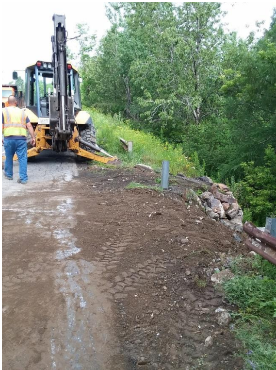
Crews working to fill in a wash area along the River Road. This wash was nearly 20 feet deep and was within 4 feet of the edge of asphalt.
