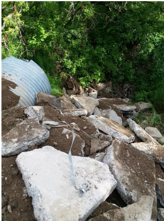
Concrete slabs from the home demolitions have been used to stabilize the wash out area and will prevent future erosion around this culvert.
