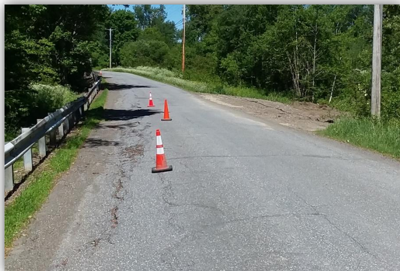
Figure 8: Portion of affected road where additional materials were placed by the city to accommodate heavy farm equipment travel.
