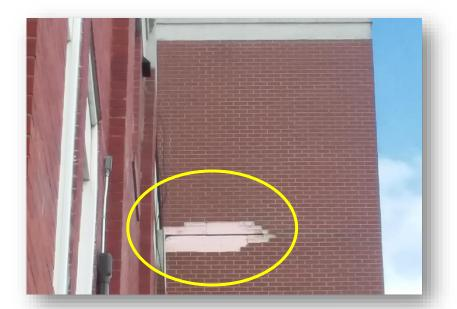
Loss of thin bricks from exterior of police station. Occurred prior to September 2015<sup>2</sup>
