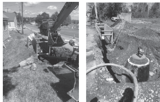
(L) Tie-in b/w Fort & Washington Streets along Route 1 (R) New manhole and 300 LF 8" sewer main, Sincock St.
