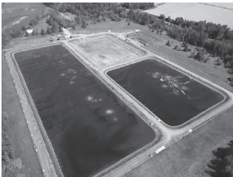
Lagoon #3; sludge removed, before new liner
