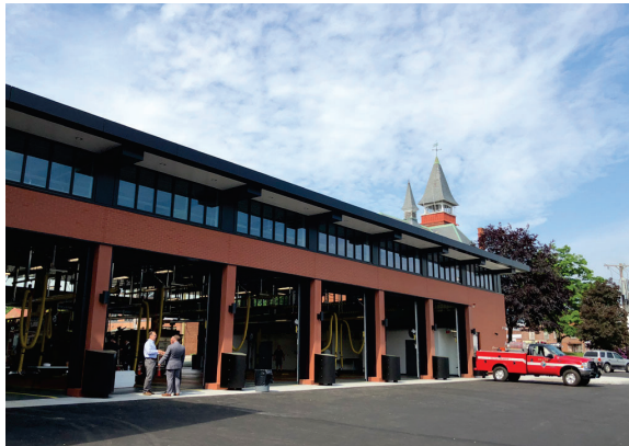
Walpole Central Fire Station
