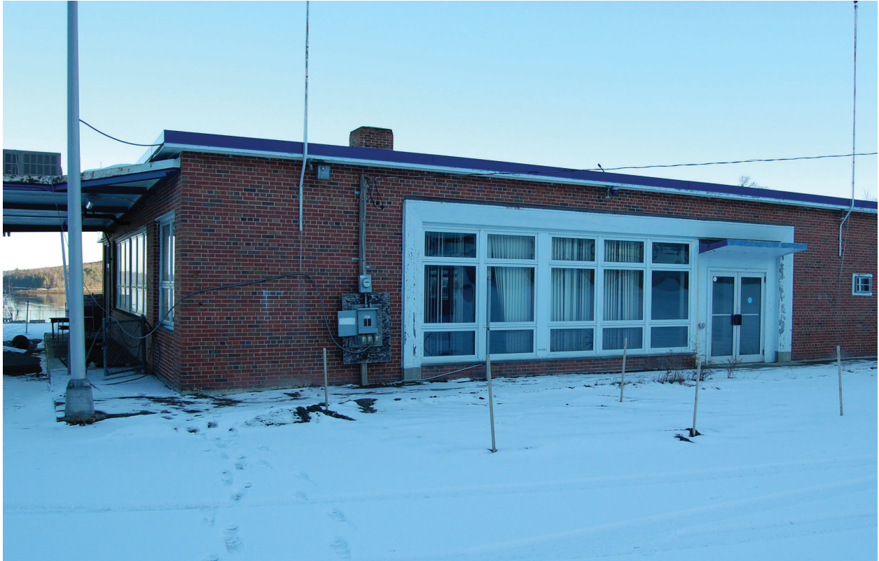
The exterior of the building prior to renovation.
