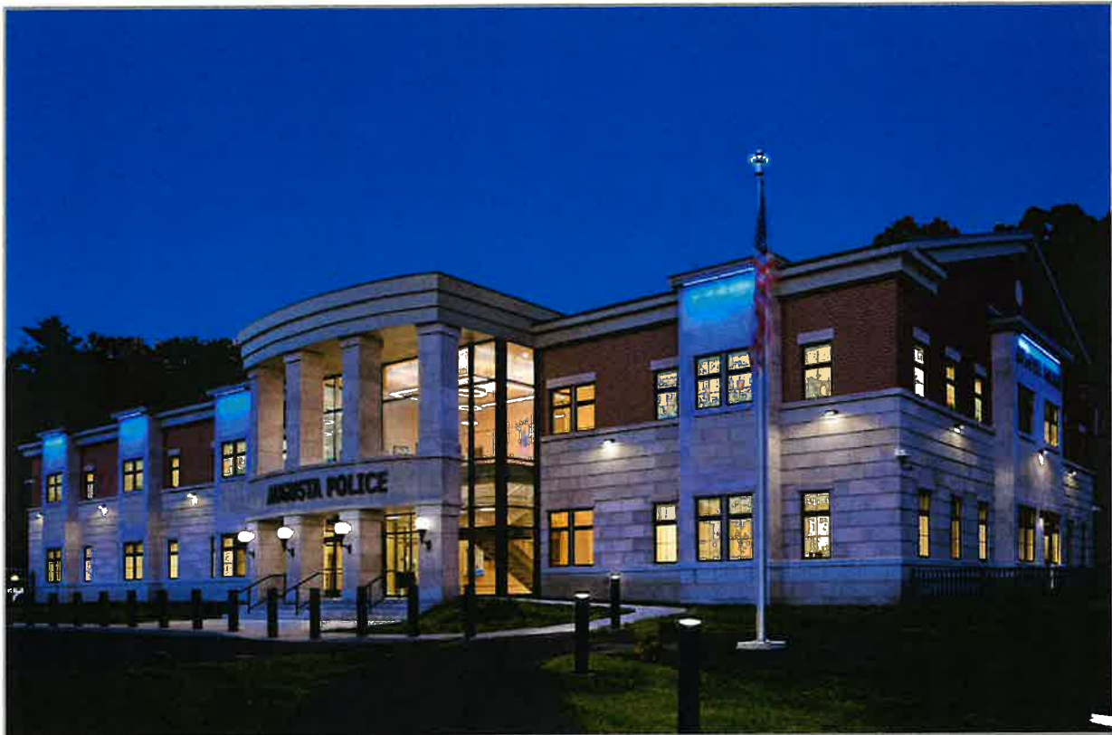
Augusta Police Station Augusta, Maine
