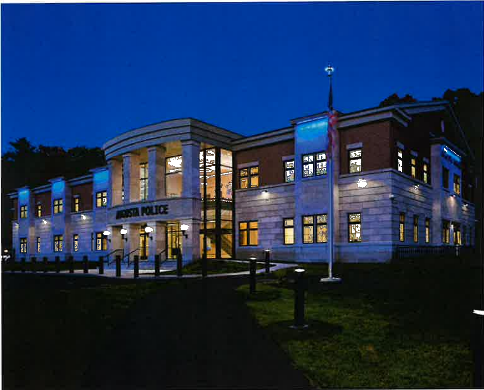
Augusta Police Station Augusta, Maine
