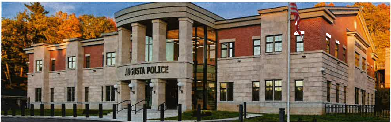
Augusta Police Station Augusta, Maine
