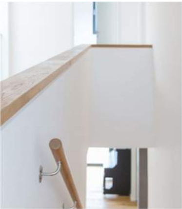
RAILING Sheetrock w/ wood cap
