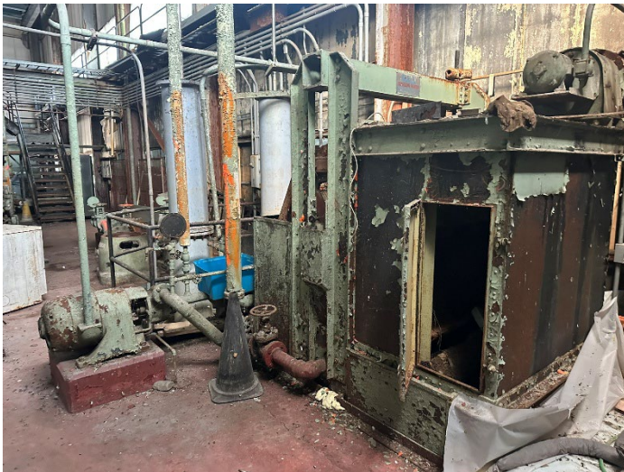
Photo 3: View inside the Steam Plant.
