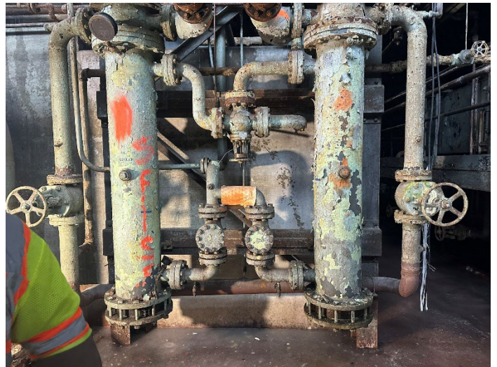
Photo 4: View inside the Steam Plant.
