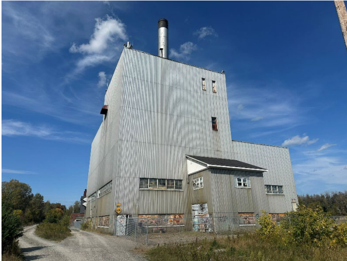
Photo 1: View of the Steam Plant- south & west sides.
