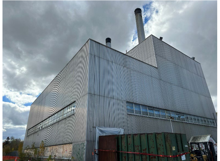
Photo 2: View of the Steam Plant- north & east sides.
