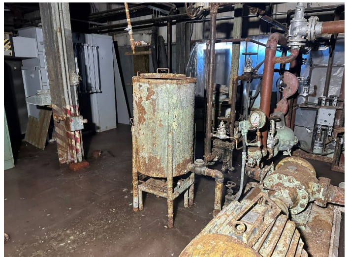
Photo 6: View inside the Steam Plant.
