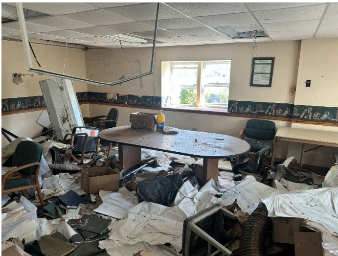
Photo 5: View inside the Steam Plant.
