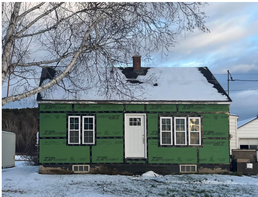
Figure 5: Updating development standards such as required setbacks, lot areas, and lot coverages ultimately increases development flexibility and lowers the cost of construction, enabling new housing.
