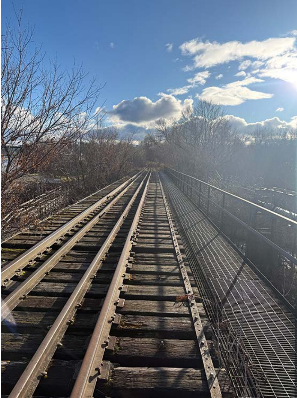
Figure 22: Existing Railroad Bridge at Caribou Stream. This City does not own this bridge or have access. Access/use discussions for the bridge and the rail corridor to continue with the State of Maine.
