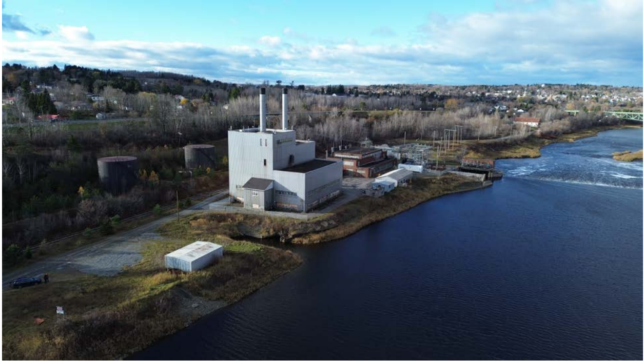
Figure 5: Existing View of Area 2 / Steam Plant Site looking Northwest
